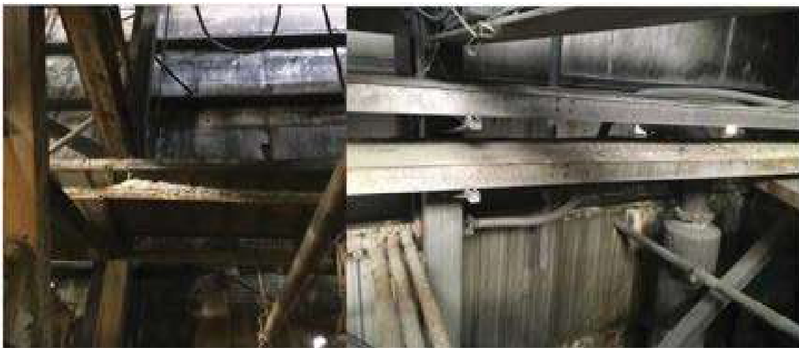
Figure 10. Cable tray's full and corroded/full of tailings.
