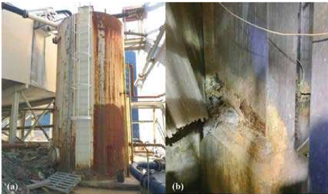
Figure 7. Examples of existing equipment corroded from contact with tailings (a) Process water tank and (b) Building column.
