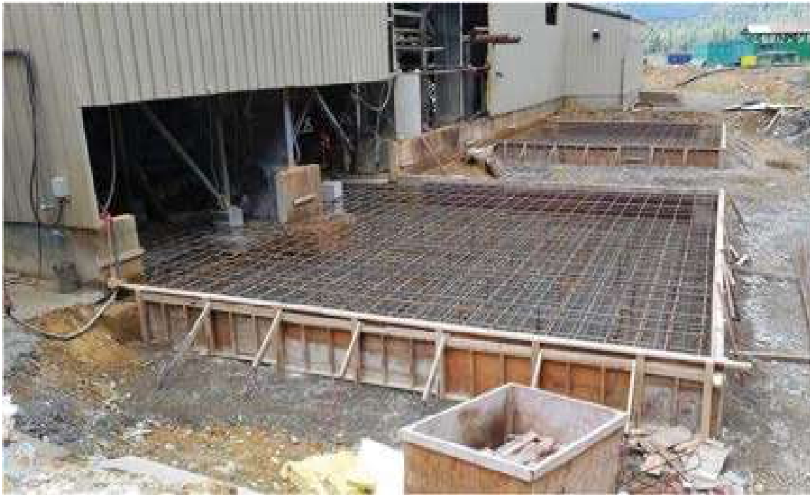
Figure 8. Silo and filter feed tank raft footings.
