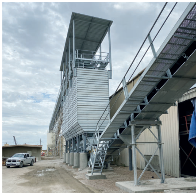
Nestled in Grand Prairie, TX – a Simem WetBeton100 aggregate loading and storage solution holding 600 tons (364 m 3 ) of material. A standard solution designed for future expansion and hot-dipped galvanized for longevity.
