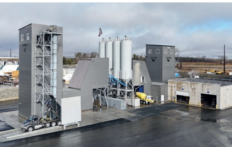
Full view of the two Simem Wetbeton WB180S plant (NEP named, the "Osprey" & Falcon")
