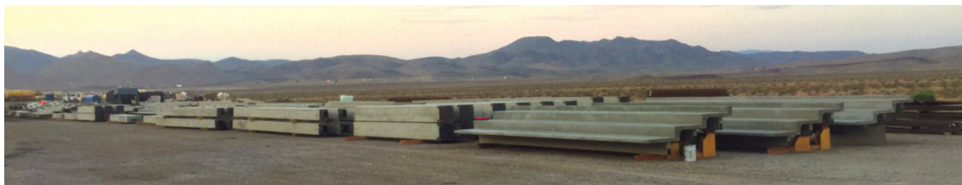
Western Pacific Precast stage the all-important stadium risers for transport, installation, and seat anchoring.
